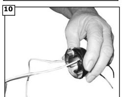
Thread leadwire and safety cable through downrod and half ball.
